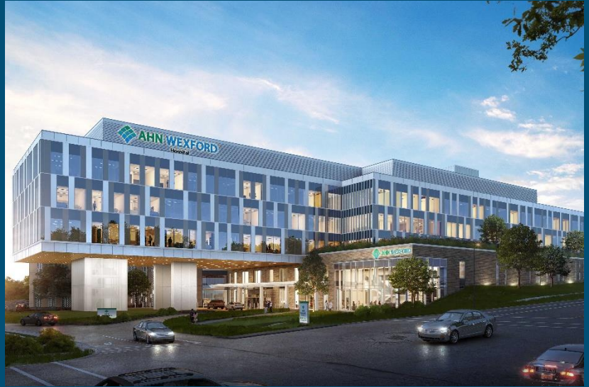
A rendering of the recently opened AHN Wexford Hospital that is home to the state-of-the-art facility with 160 beds with room to grow
